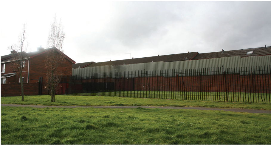
PHOTO OF EXISTING
