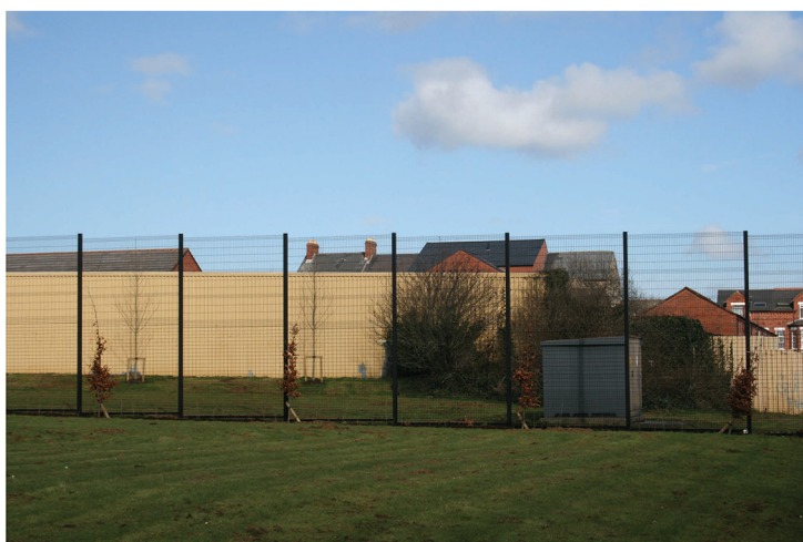
PHOTO OF SITE AFTER WORK
