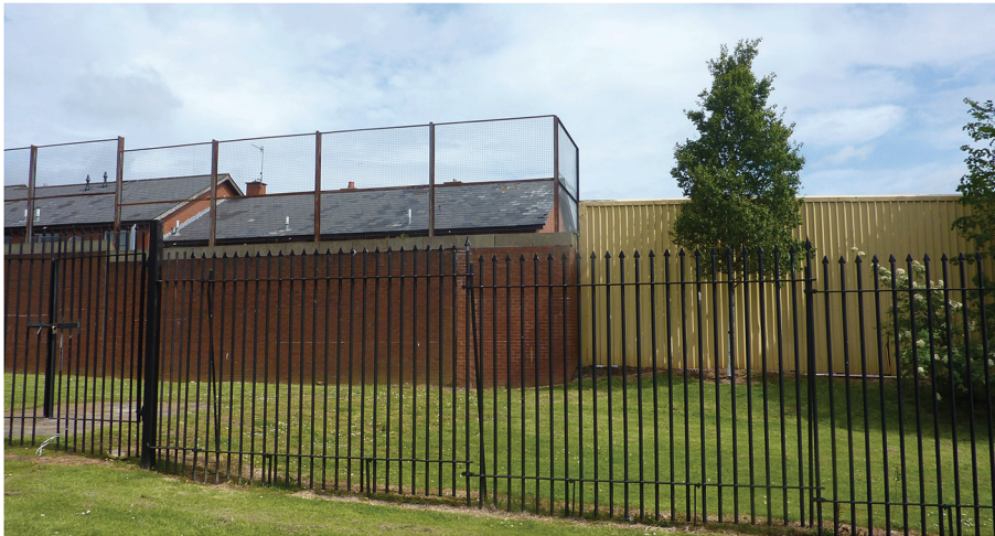
PHOTO OF SITE AFTER WORK
