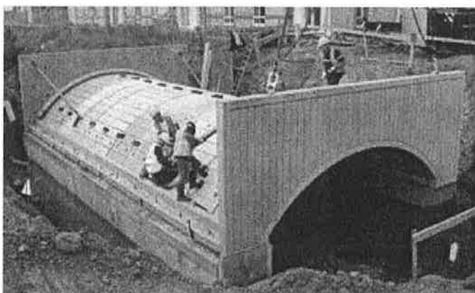
Figure 7b. Completed arch bridge before covering with backfill.
