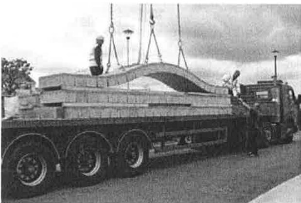
Figure 7a. Flat pack “Flexiarch” system brought to site
